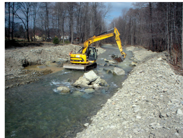
Construction in progress
