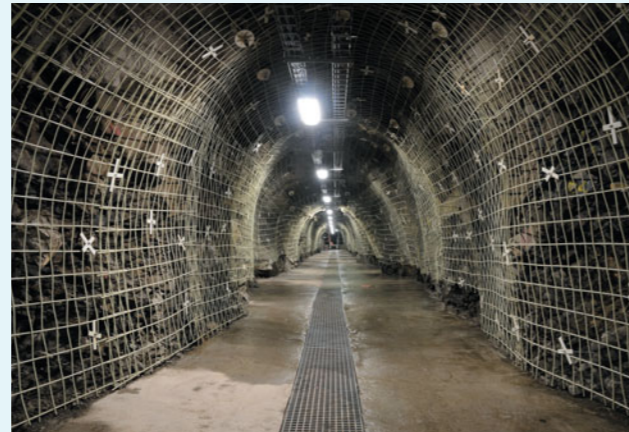
The finished draining gallery
