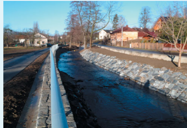
Supporting concrete wall with stone cladding running alongside the road
