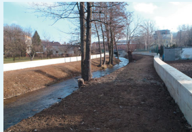
Embankment walls protecting surroundings against floods
