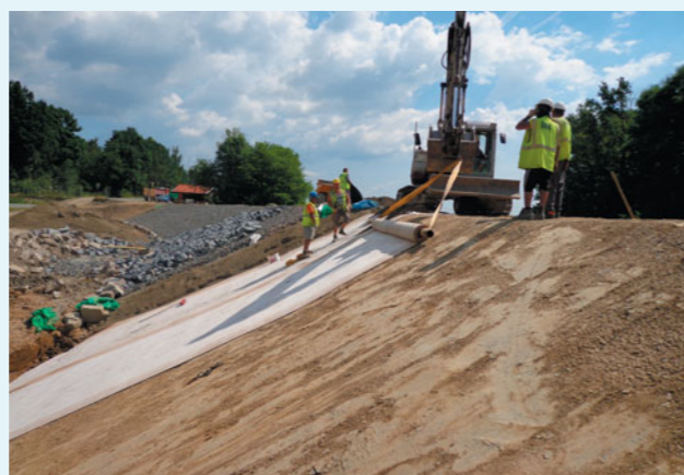
Placement of the bentonite mat
