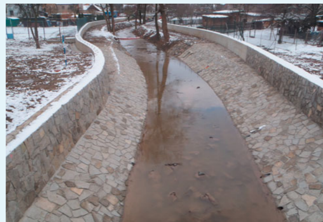
The adjusted water bed upstream of a road bridge
